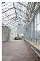
NyEi.II, Eisernes Haus, DI001518, BSV
