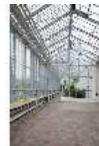
NyEi.II, Eisernes Haus, DI001515, BSV
